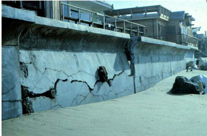
Photo 6-15. Failure of protection structure near Monterey Bay. (Source: G. Griggs)
