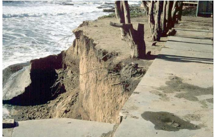
Photo 6-13. Result of wave overtopping. (Source: G. Griggs)
